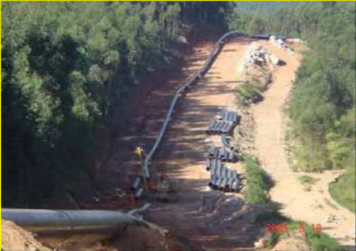
Malhas gas pipeline maintenance & gas transportation project
